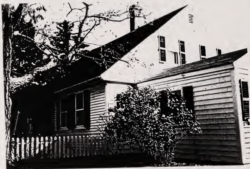
View from North
